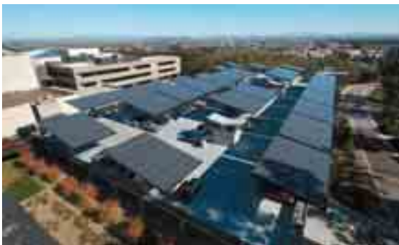
Figure 7. Hopkins Parking Structure at the UC San Diego Campus Illustrating Photovoltaic Cells for Parking Lot Canopies and High Albedo Concrete in the Driving Lanes. (vii)
