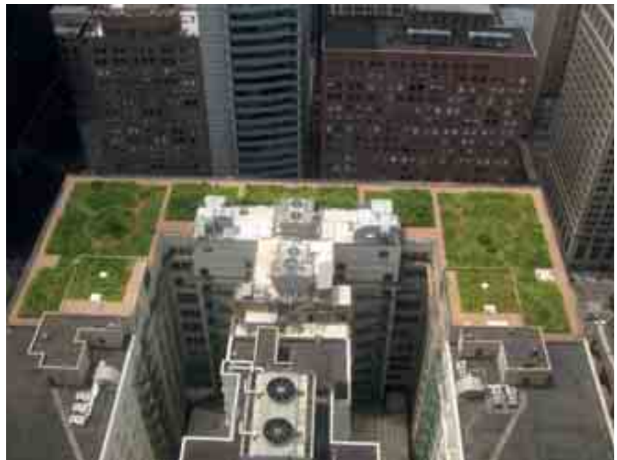
Figure 8. Green roofs like the one shown here of Chicago's City Hall, help reduce urban heat islands through evapotranspiration and reducing heat gains through the roof because of their insulating capabilities. (Source: TonyTheTiger)
